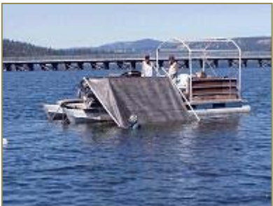
Figure 14. Installing bottom barriers
